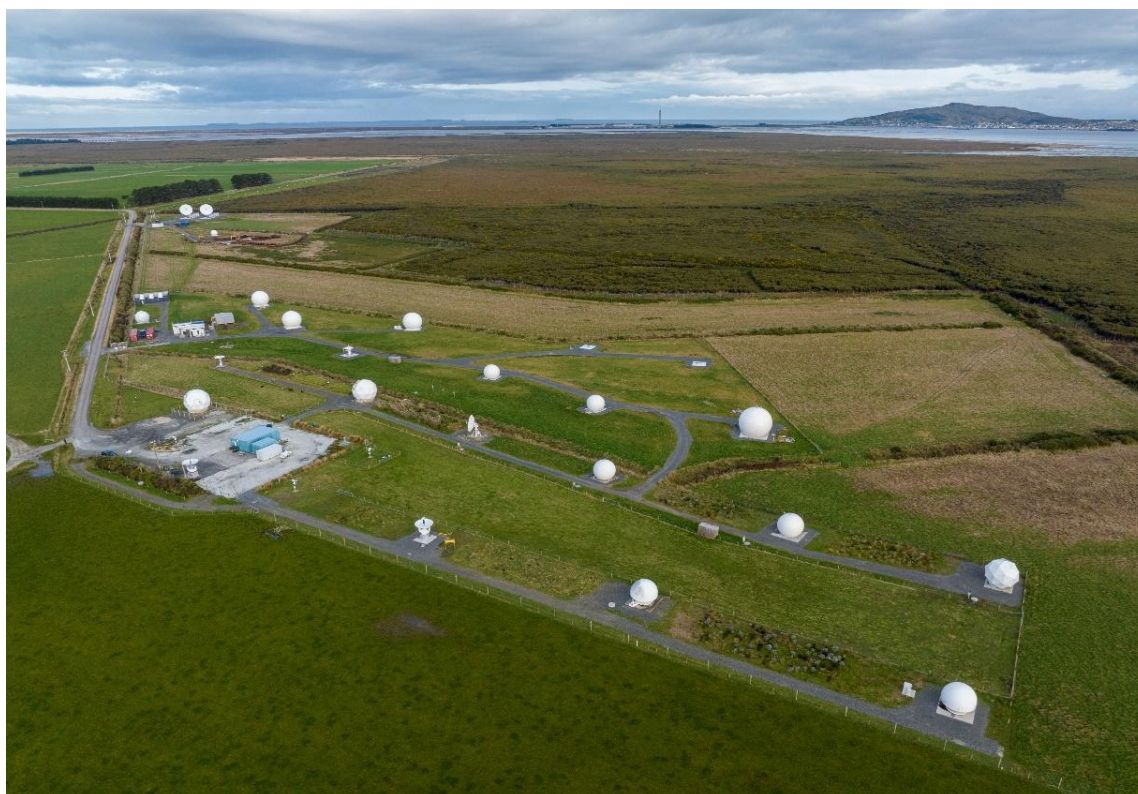
Aerial view of Awarua Satellite Ground Station
