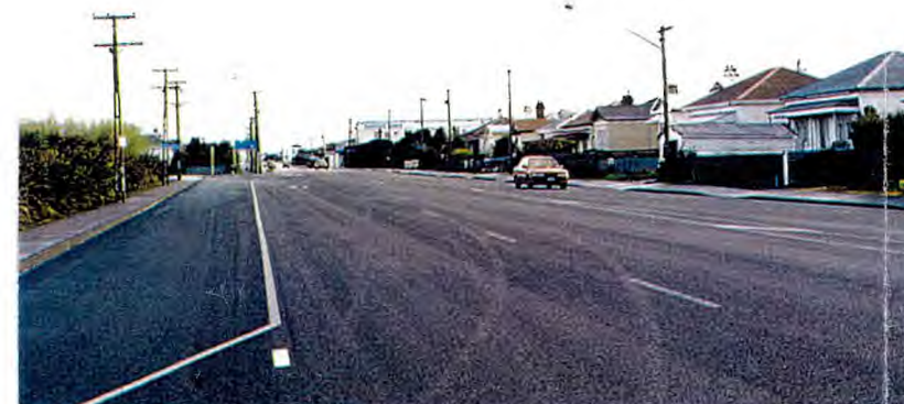
3. LOOKING NORTH ALONG ELLES RD TOWARDS SOUTHLAND TAVERN FROM KEY HOSPITAL ENTRANCE.
