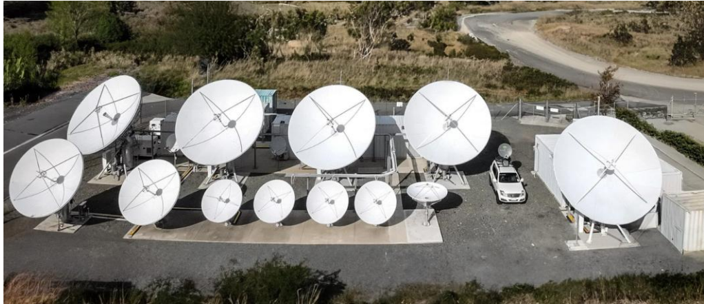
Figure 27. Gateway Teleport's ground station in Upper Hutt ( www.gatewayteleport.com ) Because the antennas communicate only with spacecraft in GEO and point in roughly the same direction as each other, the teleport requirements are relatively undemanding.
