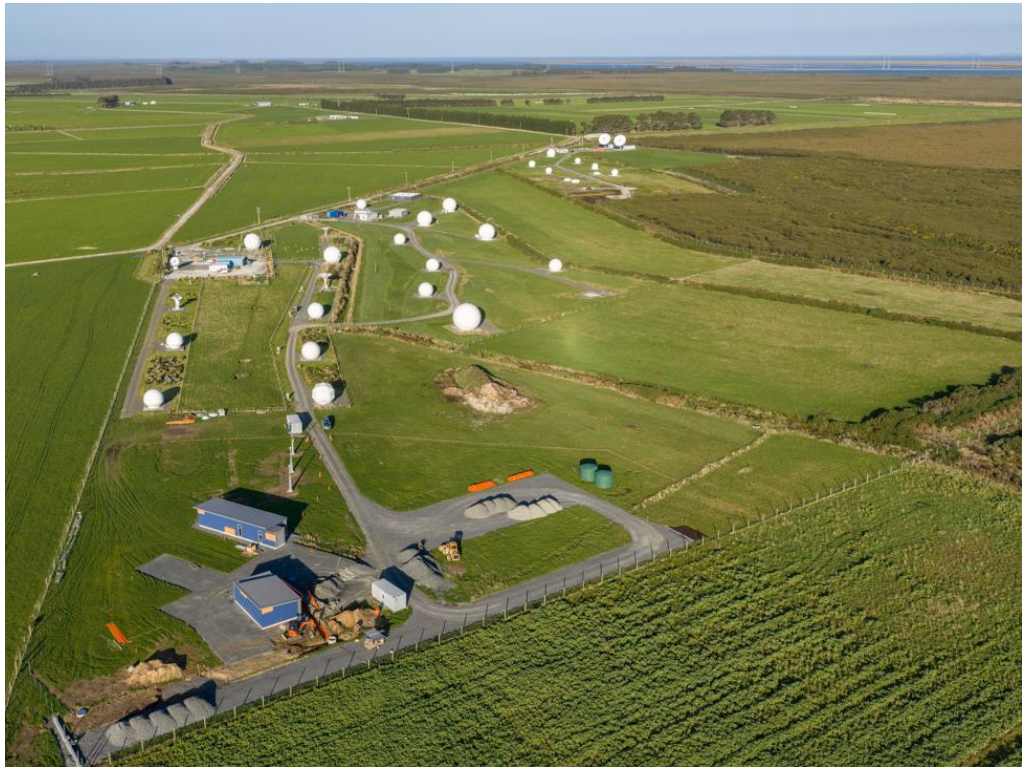
Figure 1. Awarua Satellite Ground Station, looking to the south-east, as at May 2026.
