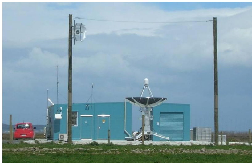
Figure 8. Awarua Station with an OTB 3.5 metre S-Band tracking antenna
