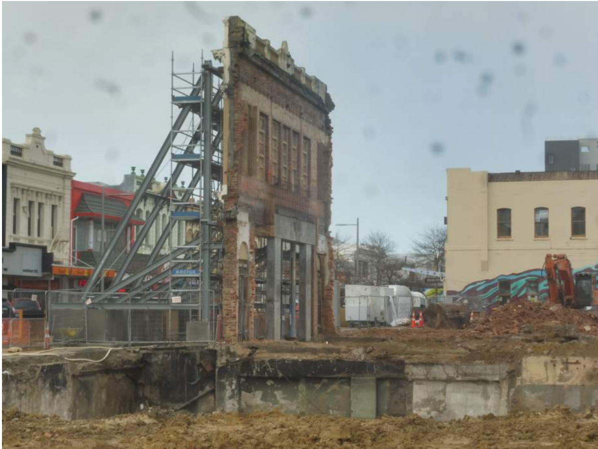
COXHEAD BUILDING FACADE RETENTION IN INVERCARGILL 2022
