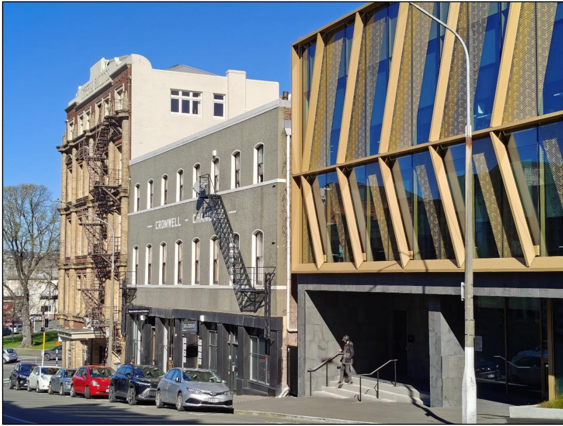
Appendix 1. The ACC building in the Moray Place – Dowling Street Heritage Precinct, Dunedin:
