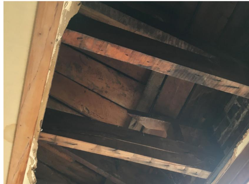
NZ native hardwood, possibly Rimu roof framing timber and sarking will be reused for specific joinery items, flooring and other interior details subject to condition.
