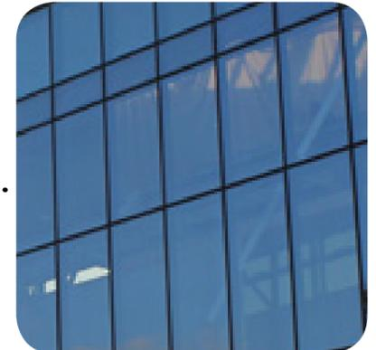
Structural glazing to provide a high degree of transparency to ground level.
