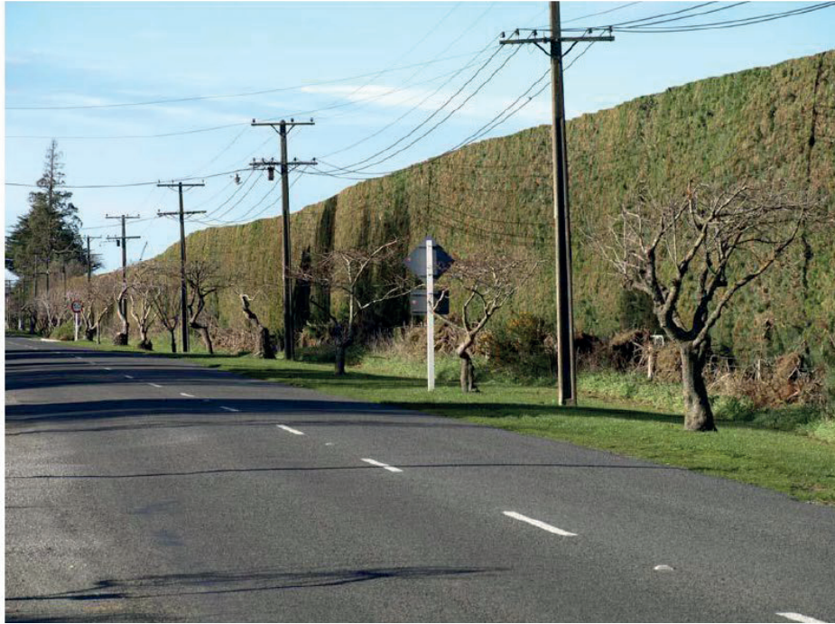
Figure 16 : Small trees planted under low and high voltage power lines
