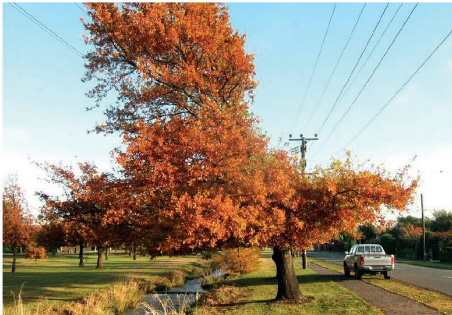
Figure 17 : Large trees planted too close to high voltage power lines
