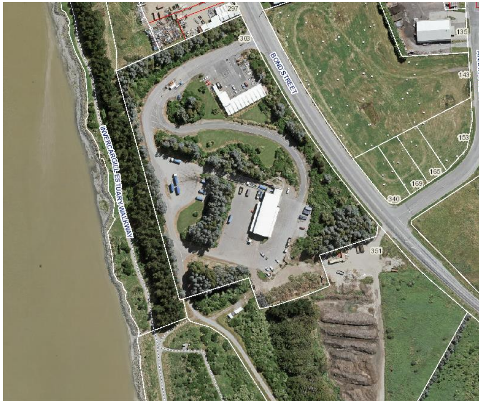
Caption: Aerial Image of Invercargill Waste Transfer Station, 303 Bond Street Invercargill.
