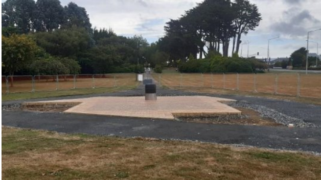
Paving installed at Umbrella Site along Town Belt, Queens Drive
